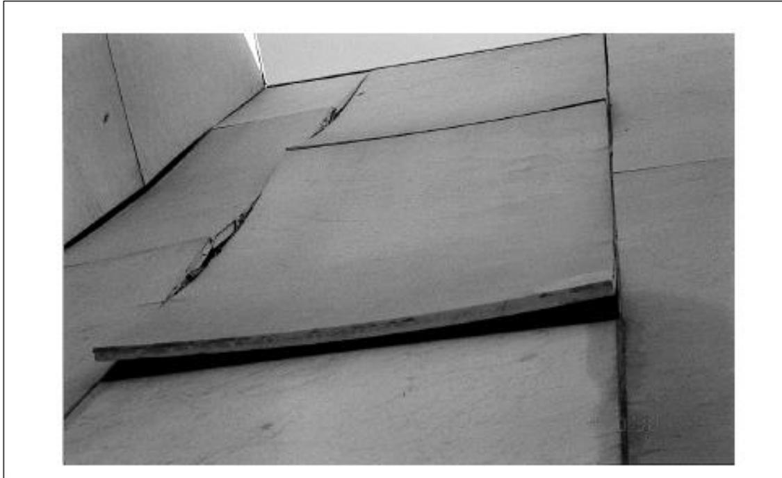
Figura1: Finland Hall in Helsinki (APRIL 1998), with evidence of bowing of the marble panels.
